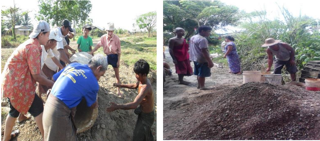
Community members repairing the road in Shwepyitha T/sp, Yangon regions
